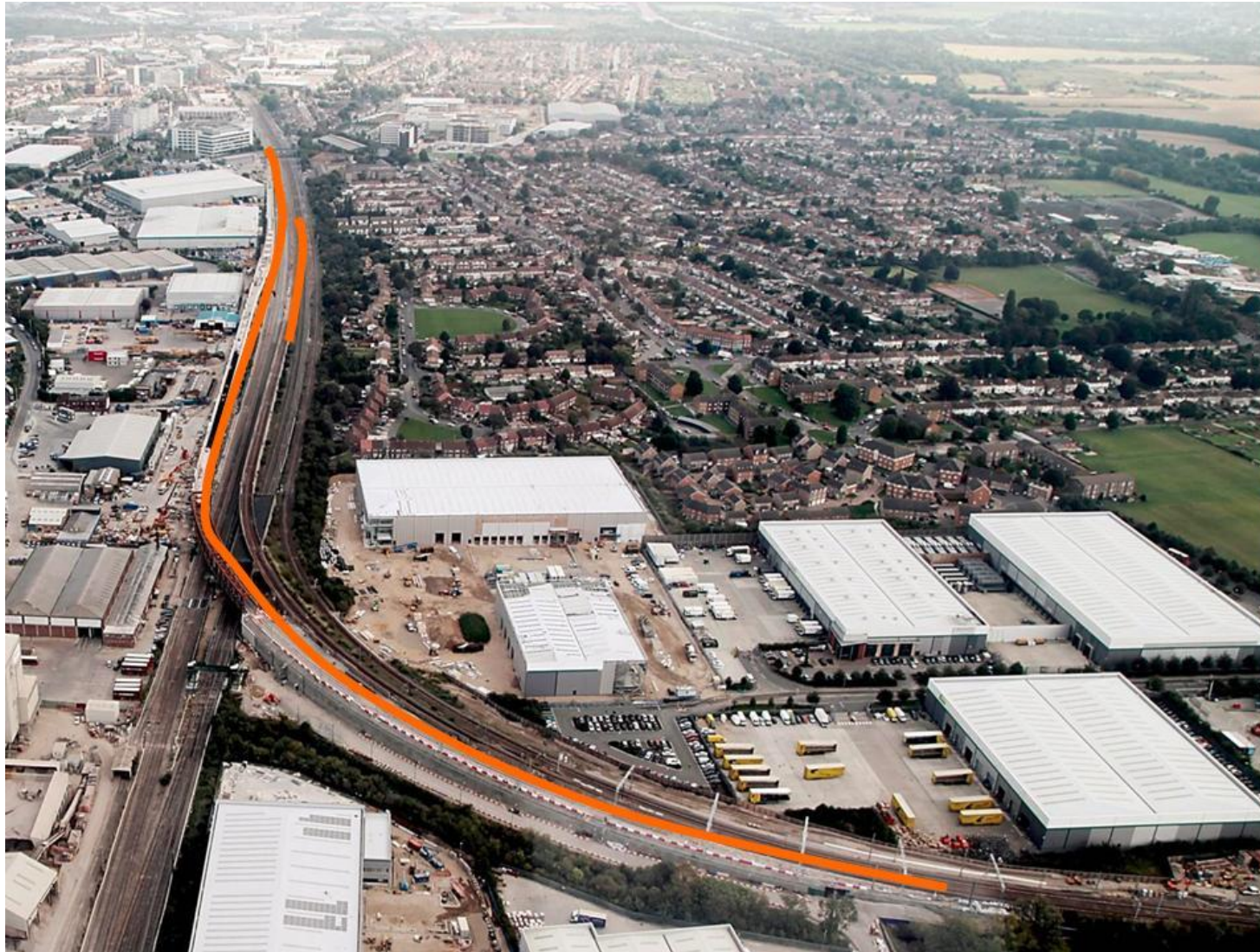
Figure 13. Stockley Airport Junction - Christmas 2014 Works
