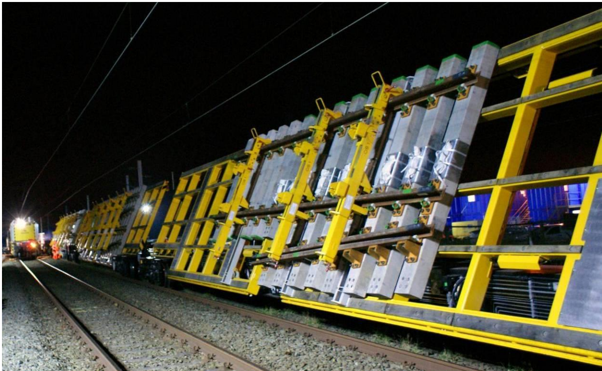
Figure 4. S&C panels ready to be lowered.
