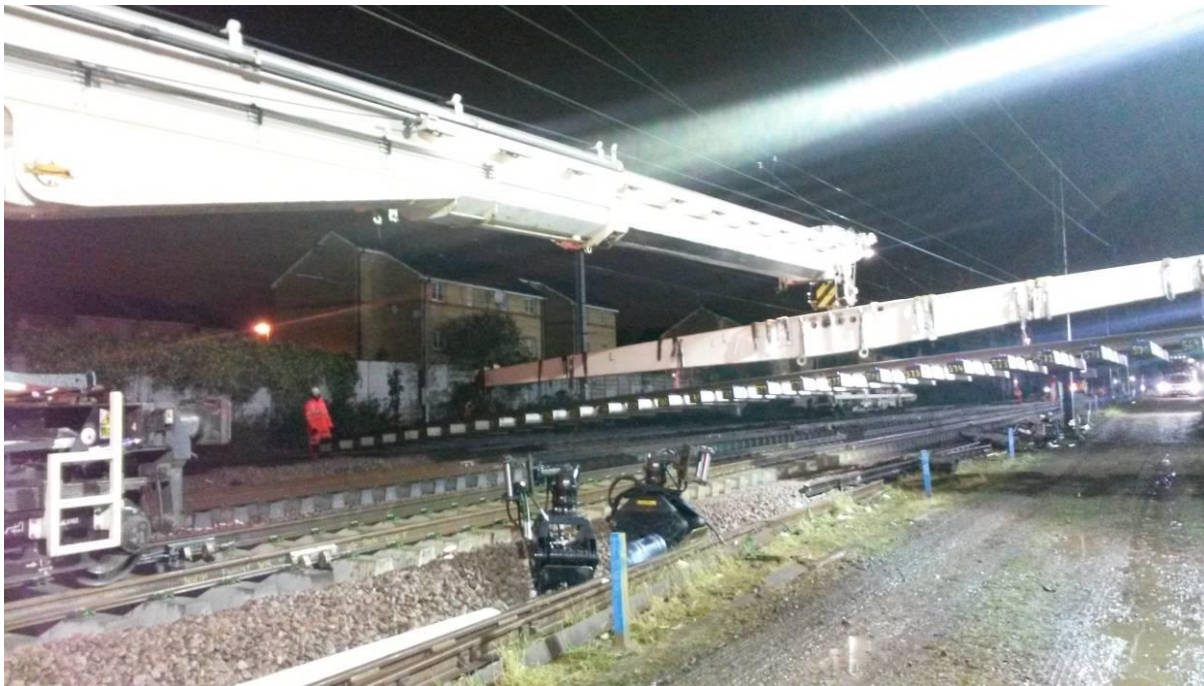
Figure 3. Above: Track panel being installed at Holloway Junction.
